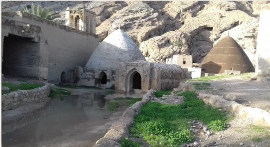
Figure 3. A photo of the reservoirs in the old village in Larestan city, captured by the author. In the northern Persian Gulf, due to drought and scarce drinking water, residents depend on reservoirs. They also diligently maintain and adhere to strict hygiene protocols, including water purification and chlorination. (Photo is taken by the author)
