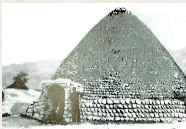
Figure 1. Exterior View of the Water Reservoir (Nabipour, 2007, p. 98)
